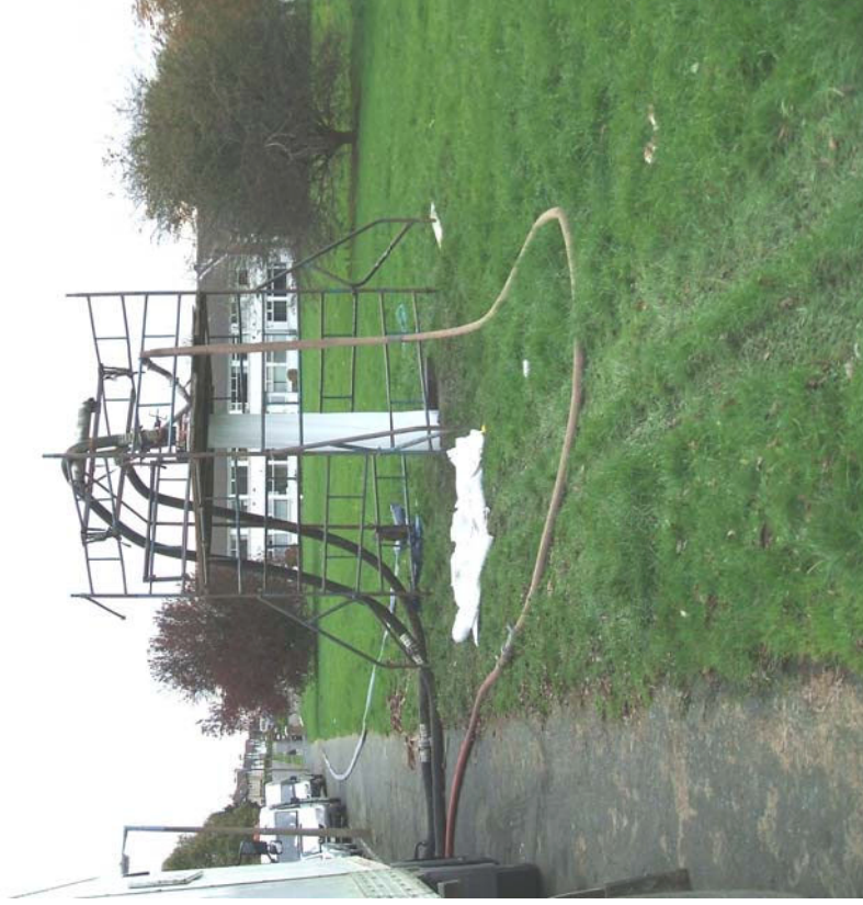
Rig set up for hot cured resin lining of culvert at High Moor Avenue (Moortown)
