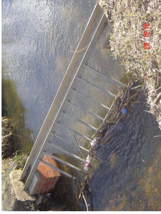
Wyke Beck trash screen (above) and Fearnville cut-off drain (below)
