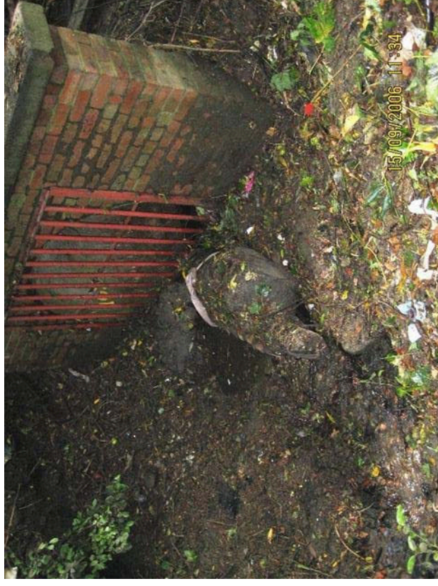
Tree trunks removed from under bridge on the River Wharfe at Wetherby (sawn into sections ready for removal)
